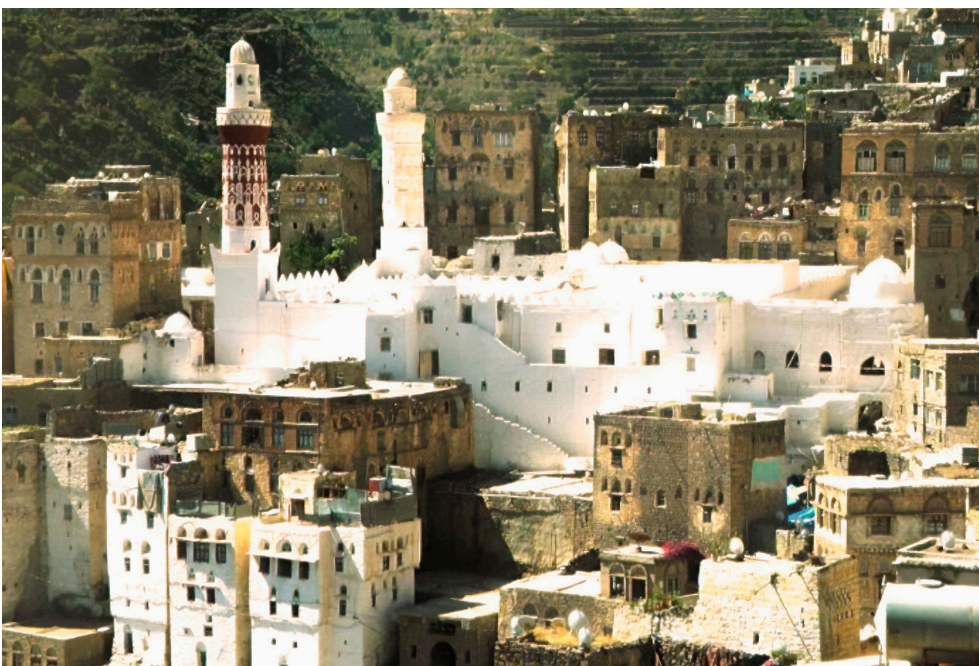
Figure 12 General view of the Great Mosque in Jiblah. Source: Al-Shehab (2024, p. 102).
